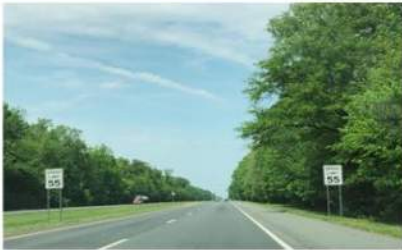
EB DE 99 (phase 2) north of 2nd St (about 0.1 miles west of Main St)
