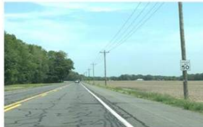
SB Main St (phase 4) west of DE 12 (about 0.5 miles north of DE 99)
